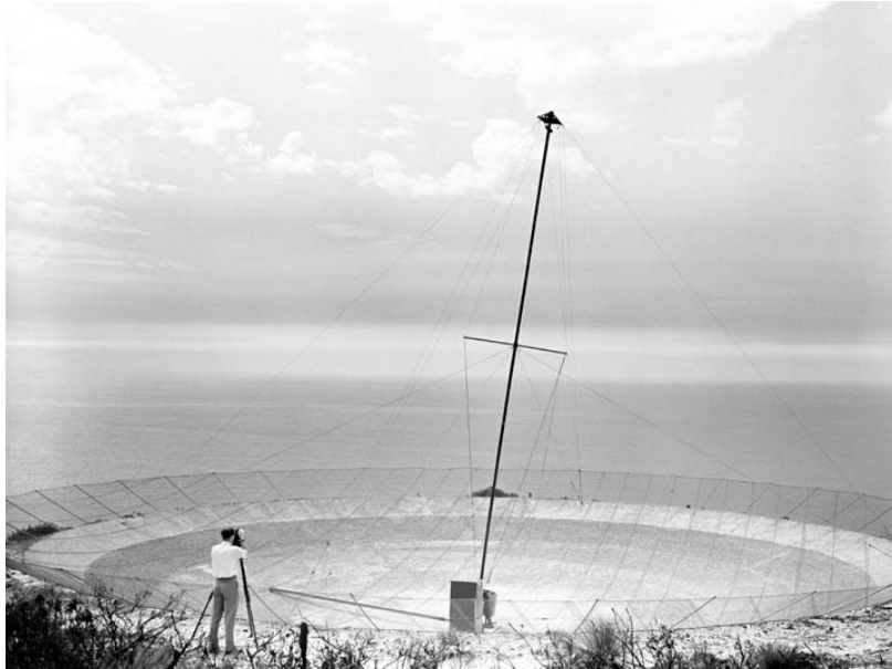
Fig. 1.1.10: Taken from CSIRO Gordon Stanley is seen using a theodolite to pinpoint the position of the antenna mast. This radio telescope was used to survey the sky for radio sources, and for a detailed study of a strong radio source that was detected in the constellation of Sagittarius. The radio astronomers realised that this source (called Sagittarius A) was located at the very centre of our Galaxy! These observations gained further fame for Australia and Dover Heights when in 1958 the International Astronomical Union decided to adopt the position of Sagittarius A as the coordinate centre for the system of galactic 'latitude' and 'longitude' that is still used today by all astronomers.
